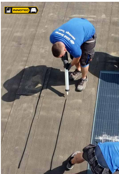
Applying the Innotec adhesive
