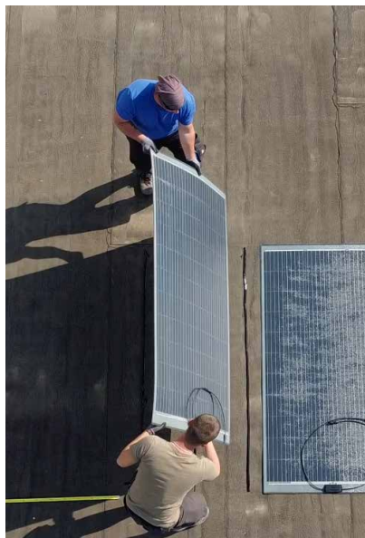
The DAS Energy modules are bonded directly to the substrate.
