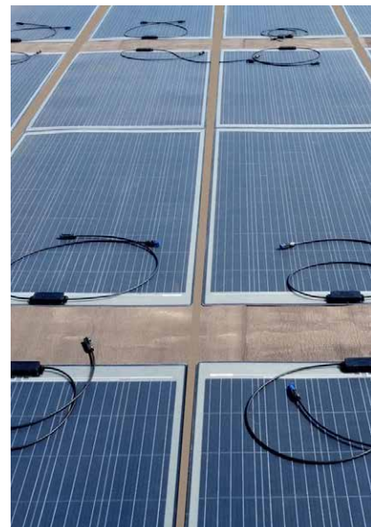
DAS Energy modules mounted on bitumen
